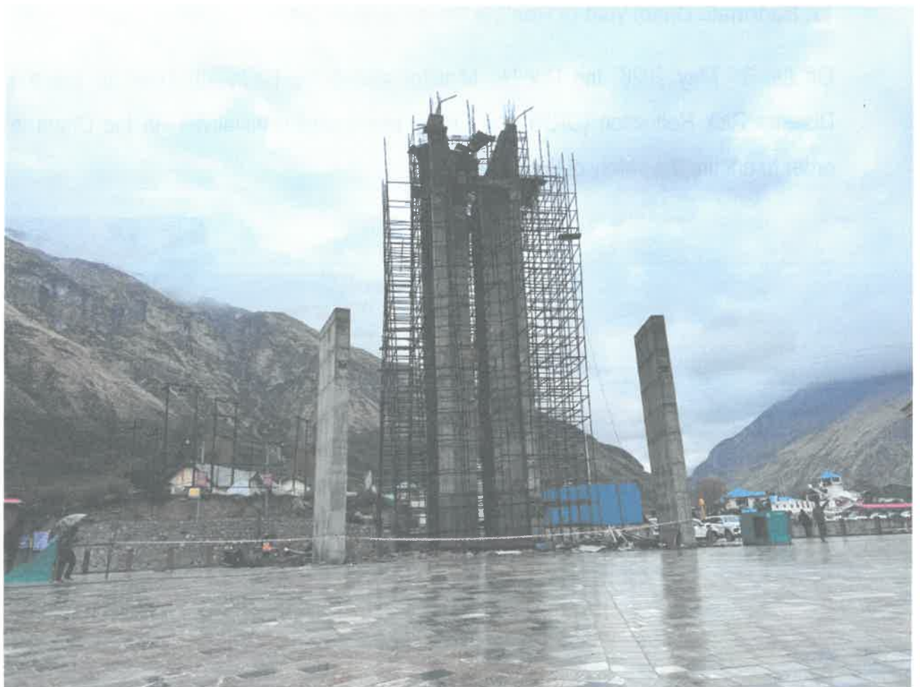
Clock Tower coming up at Badrinath Dham complex.
