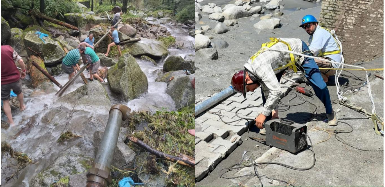
Restoration Work of WSS Schemes
