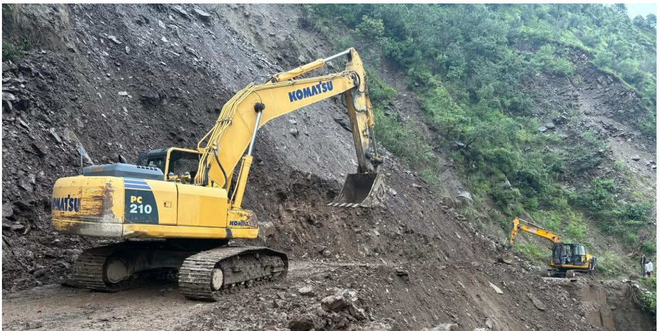
Restortaion of NH154A in District Chamba
