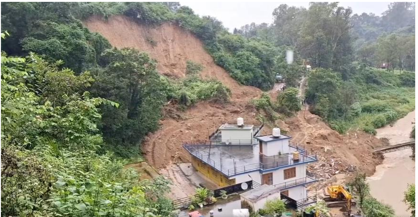
Landslide site at Sundernagar
