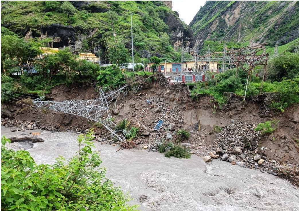
Figure 3. One 66 KV Double Circuit Transmission Tower is damaged near power House of Stage-I
