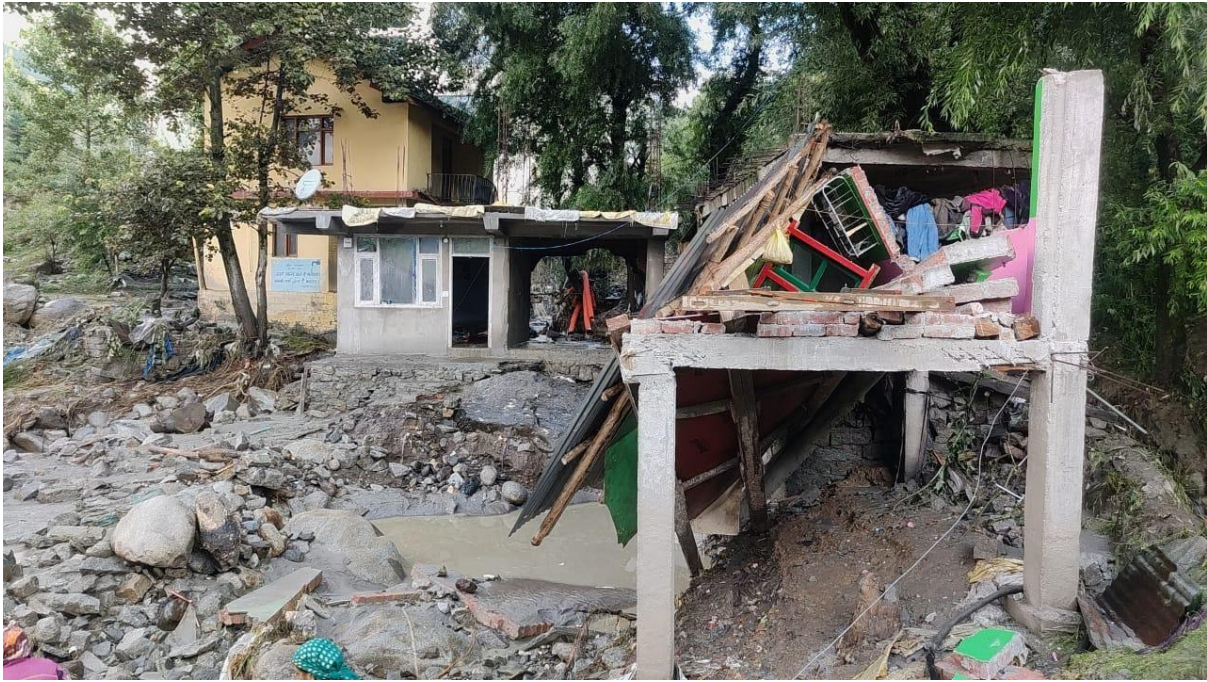
Damage to local residents
