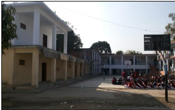
Fig.5 Vertical irregularity
