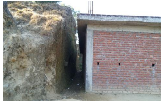
Fig.16 inappropriate distance between cut slope and building wall (GPS Panyala)
