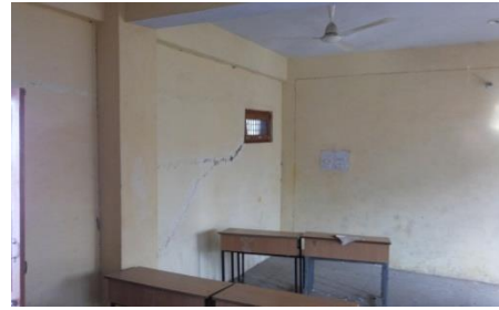
Fig.14 Incorrect ventilator placement (GSSS Tal)
