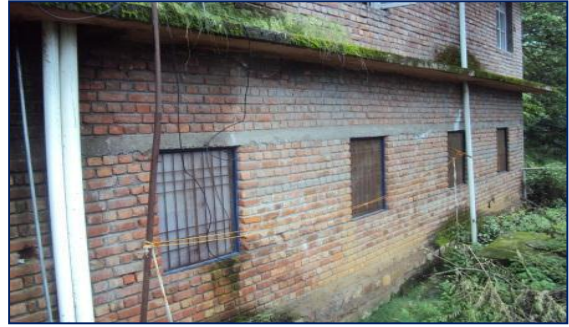
Fig. 4 plinth band and roof band
