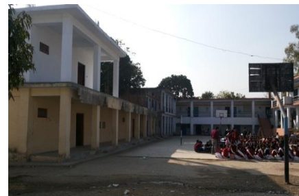
Fig.12 Vertical and plan irregularity(GSSS Tal)
