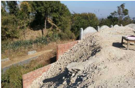
Fig.15 Inappropriate construction practice boundry wall acting as retaining wall
