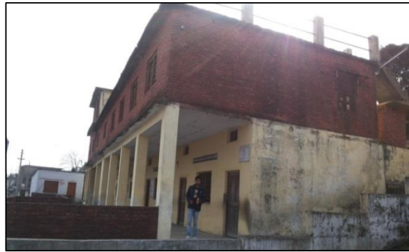
Fig.6 Mass irregularity
