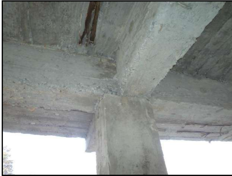
Figure 28: Wrong Practice of Beam Column Junction
