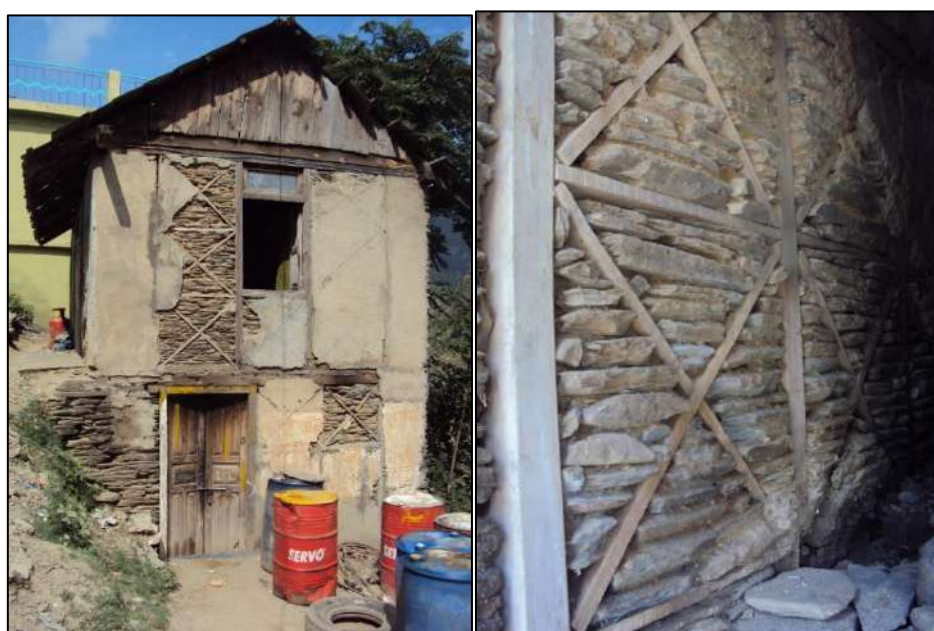
Figure 19: Dhajji Dewari Type House (Shimla, 13 th November 2013)
