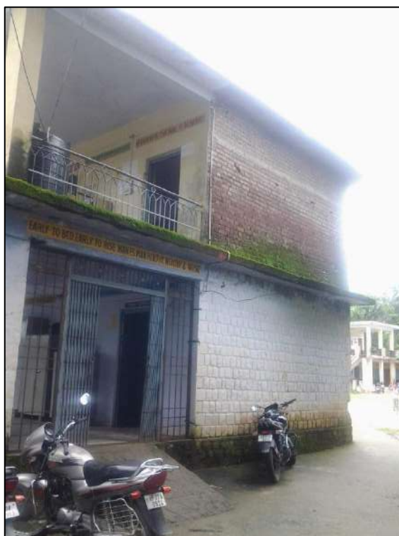
Figure 25: Hybrid Construction (Stone masonry and brick masonry)
