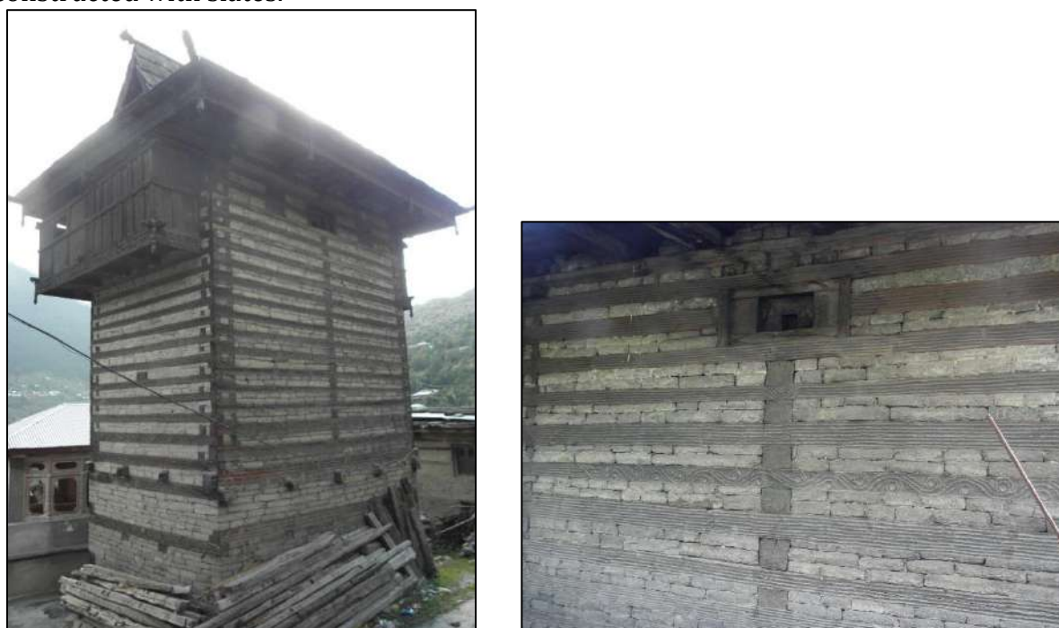
Figure 21: Kath Khuni Architecture (Village: Dharmaling, Kinnaur, 29th September 2013)
